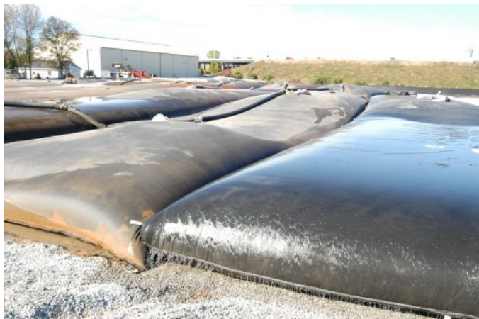
Photo 10: Geotubes (note one Geotube in the process of dewatering)
