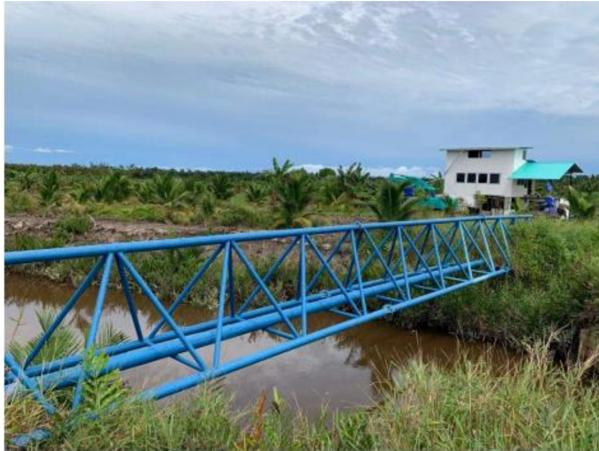
Pipe Bridge Kg. Semawang
