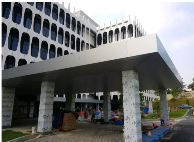
Blok MP – Covered walkway / porch
