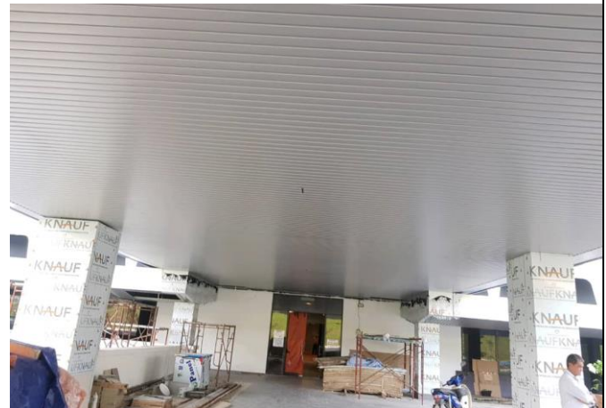
Blok MP – Covered walkway / porch
