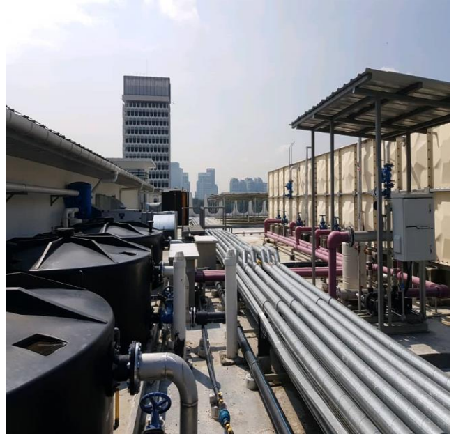
Aras lift motor
