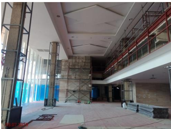
Aras Tanah – Main Lobby
