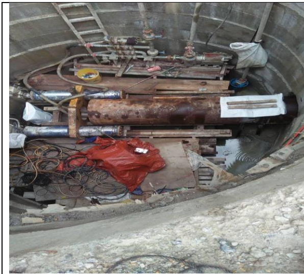
MH5 –MH5S – MH6s – Manshield pipe sleeve jacking
