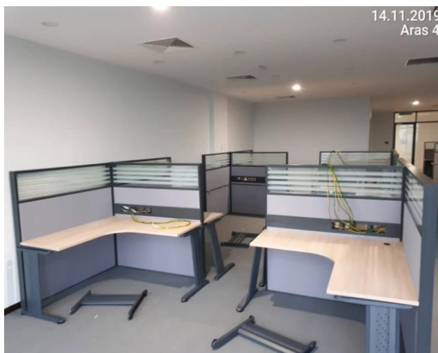
Aras 4 – Pemasangan workstation
