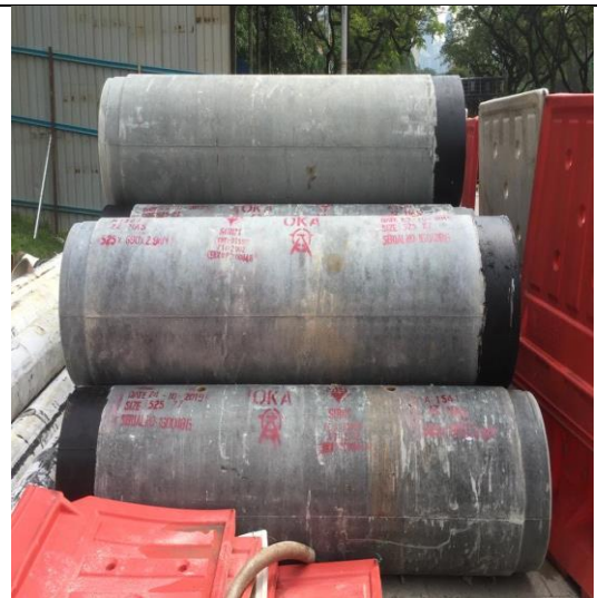
MH5 –MH5S – MH6s – 525mmDia RC pipe
