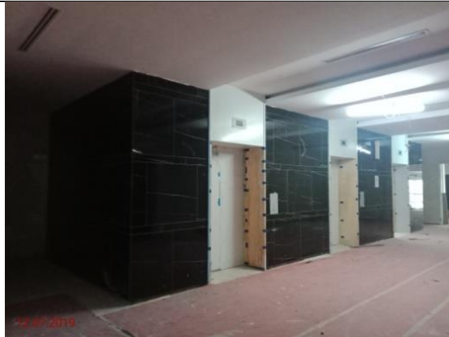
Aras 1 - Lobby Lift
