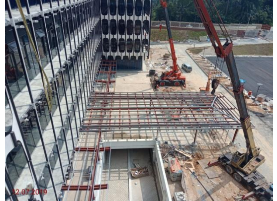
Covered Walkway Blok MP
